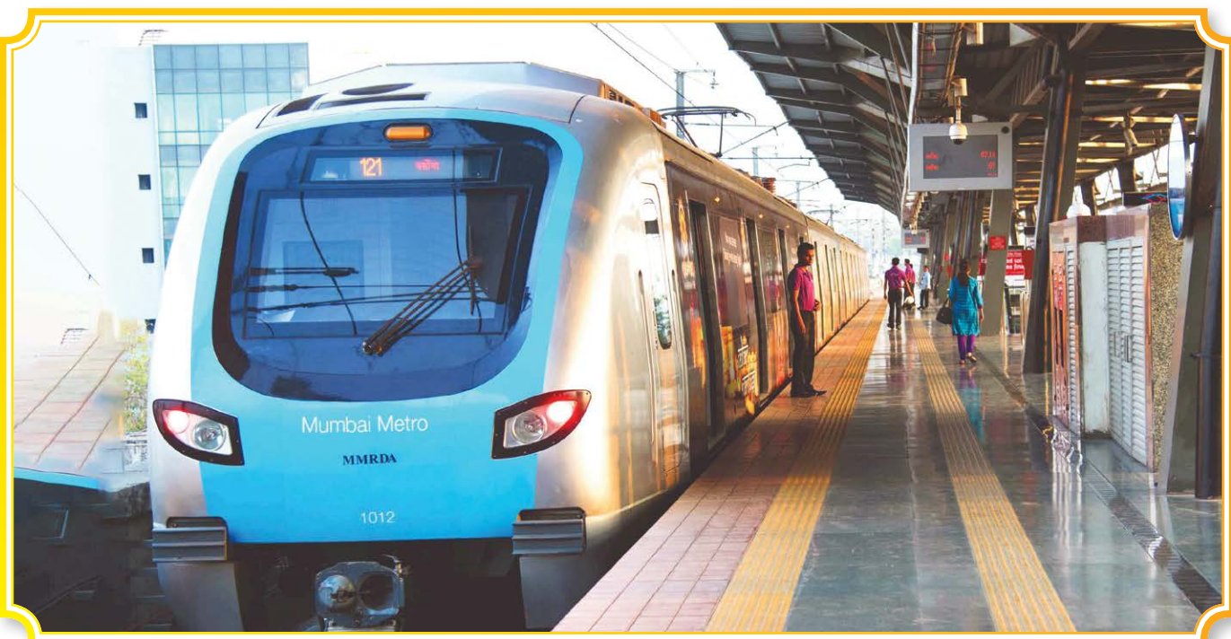
Mumbai Metro Project financed by REC
